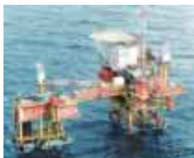
Four Crude oil pumps in the North Sea (Dual Voltage 2300-3300V / 160A)
